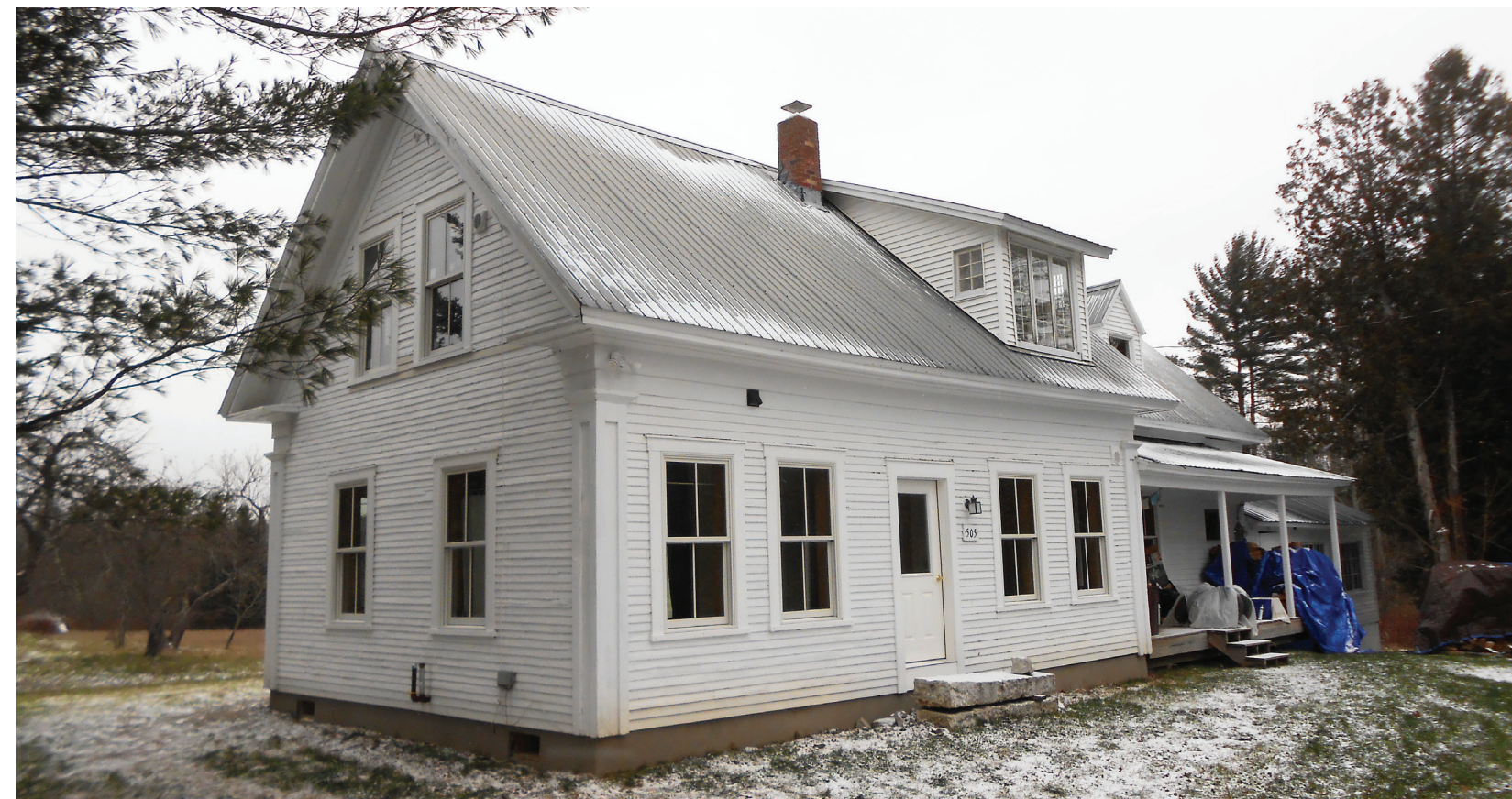
Efficiency upgrades turned this once-uninhabitable Greensboro farmhouse into a cozy home in 2017.
