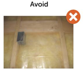
Insulation compressed behind electrical box
