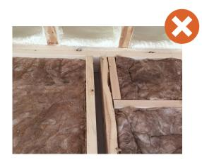
Highly compressed insulation throughout cavity, and missing altogether in some areas
