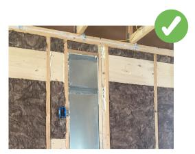
Well-detailed fiberglass, caulk/foam between narrow stud gaps
