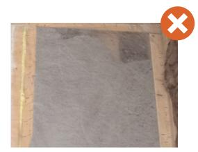
In addition to not having complete fill, the dense-pack fill is not dense enough which means it will settle even more over time
