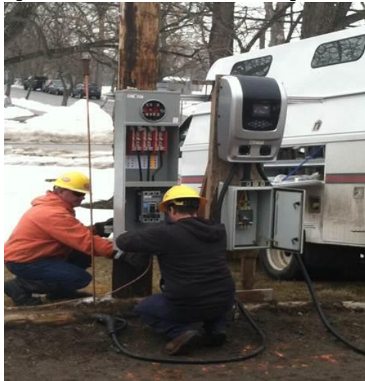
Figure 4: Installation of the EVSE at Burlington Electric
