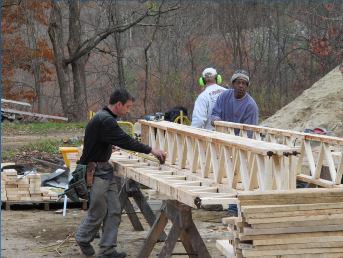
Triform joists being used as rafters. Photo: Alex Wilson
