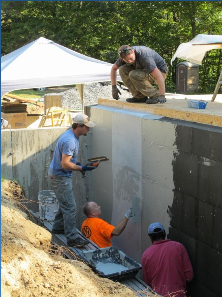
Ardicote polymer cement waterproofing layer applied to Foamglas. Photos: Alex Wilson
