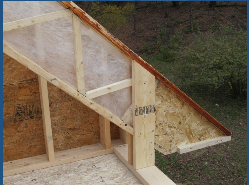
Triforce joists being used as rafters. Photo: Alex Wilson
