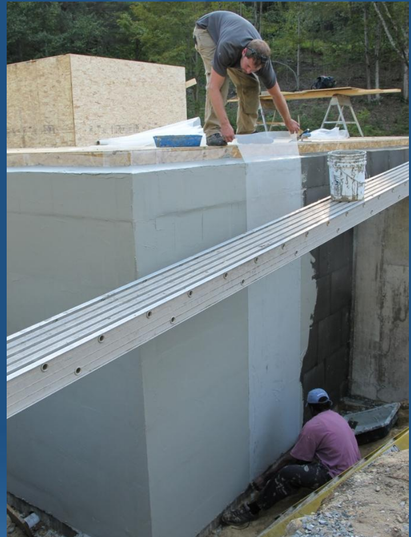
Ardicote polymer cement waterproofing layer applied to Foamglas. Photos: Alex Wilson
