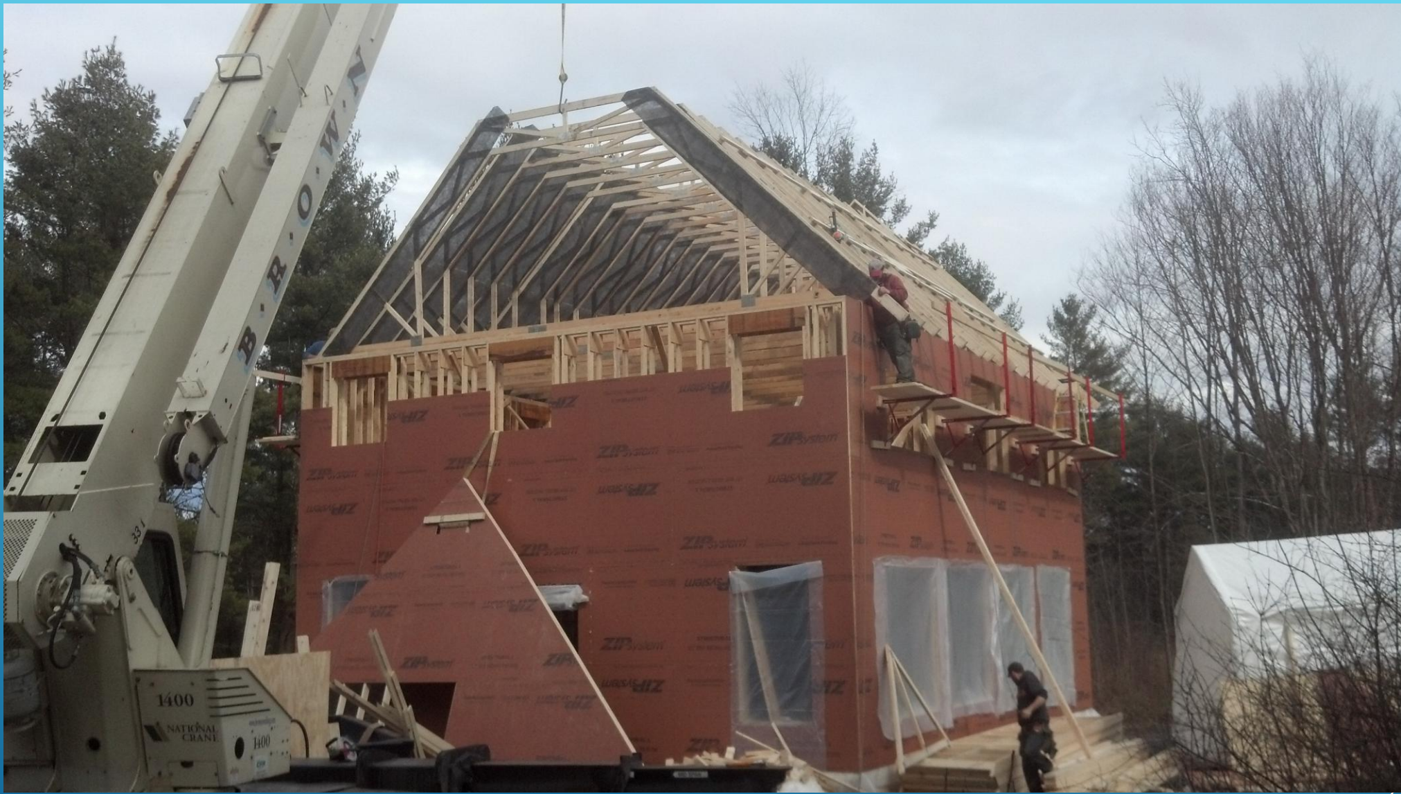
ROOF WITH ATTIC INSIDE ENVELOPE TRUSSES PREPPED FOR INSULATION
