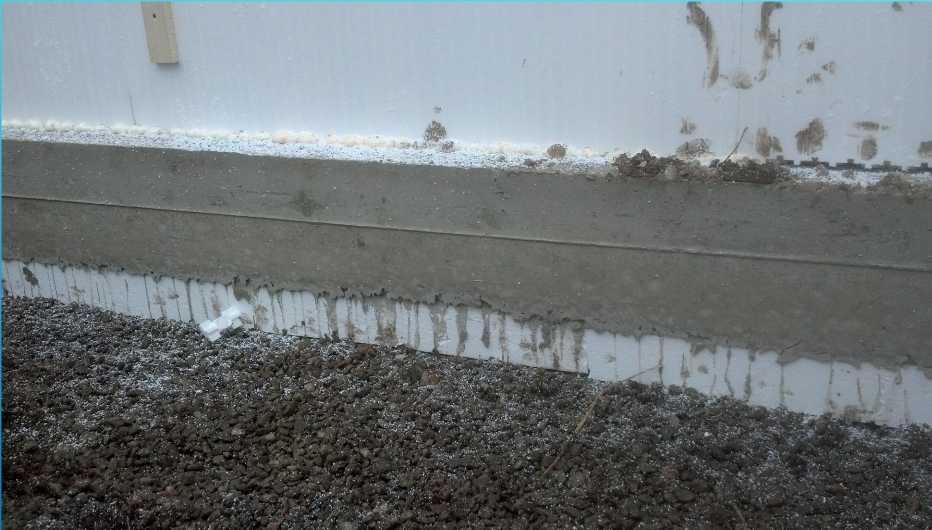
INSULATED FOOTING WITH HIGH DENSITY EPS FOAM
