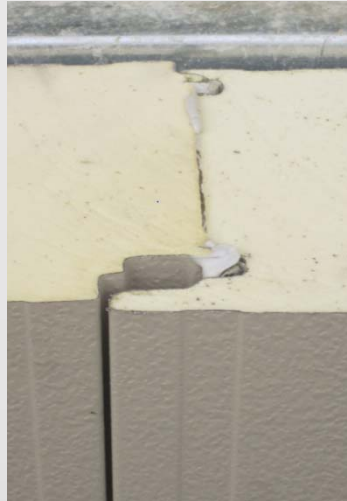
6" Insulated Metal Panel: joint detail with sealant at both tongues
