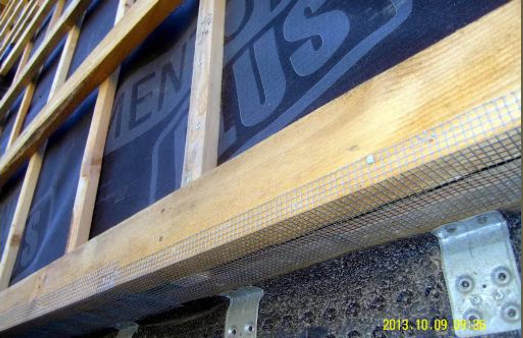
Fly Battens and wall rain plane vent
