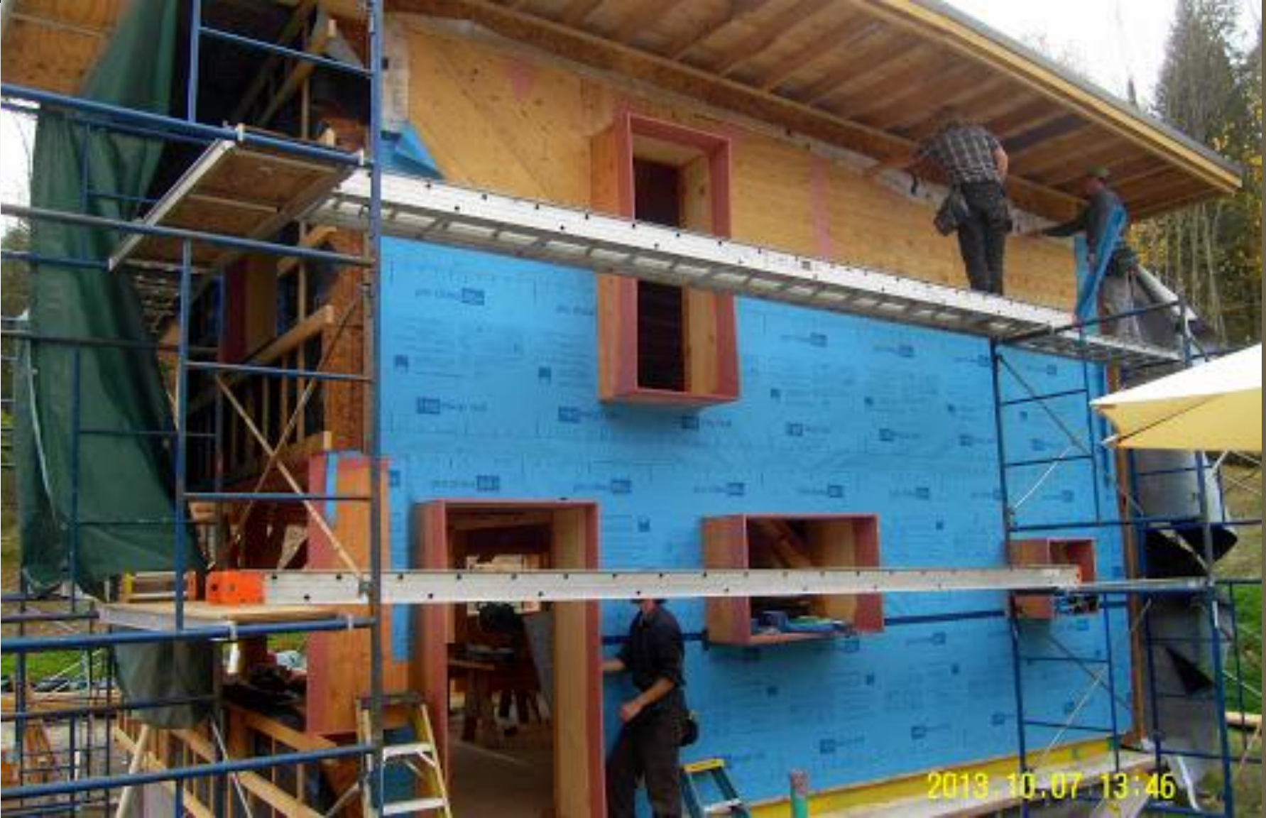
Working up the east wall
