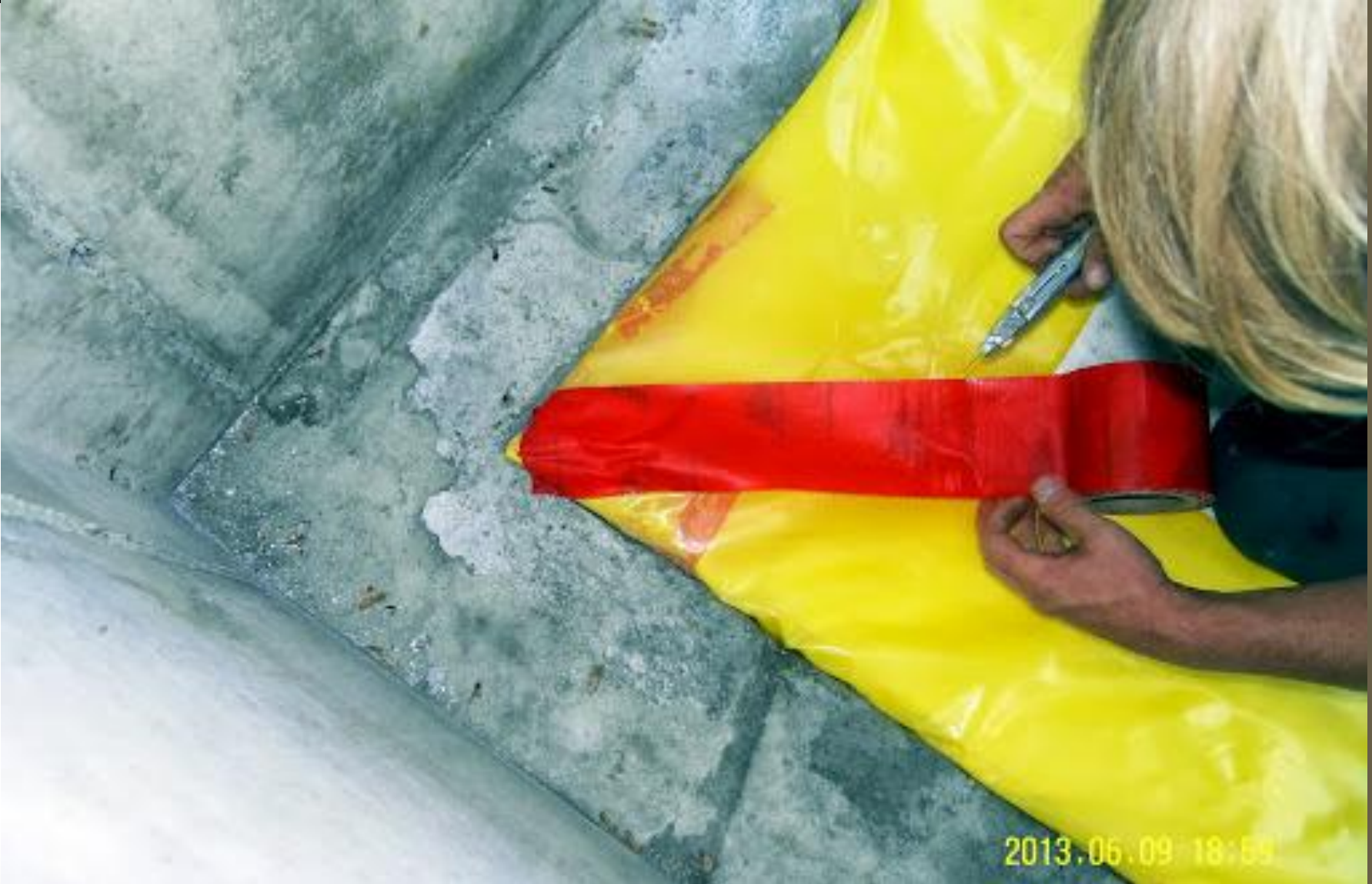
Footing AB Taping
