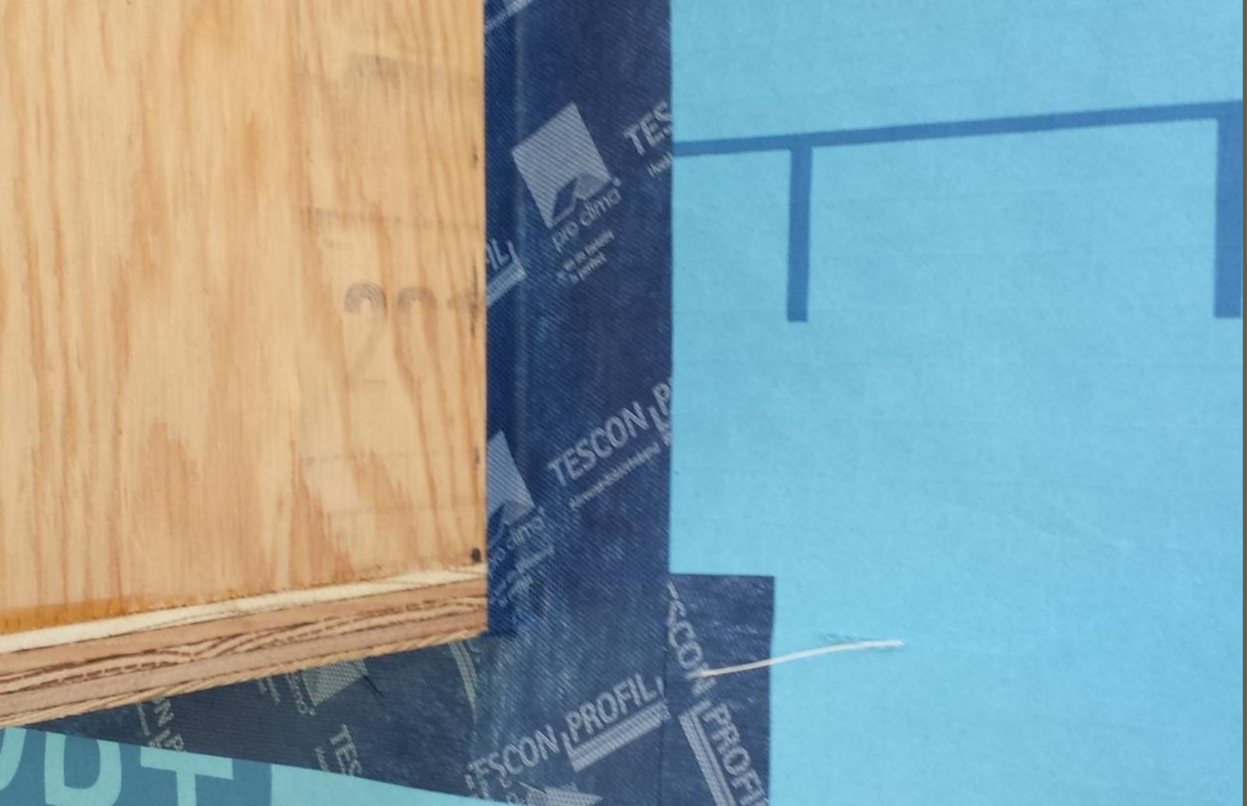
AB Air seal taped to window bucks
