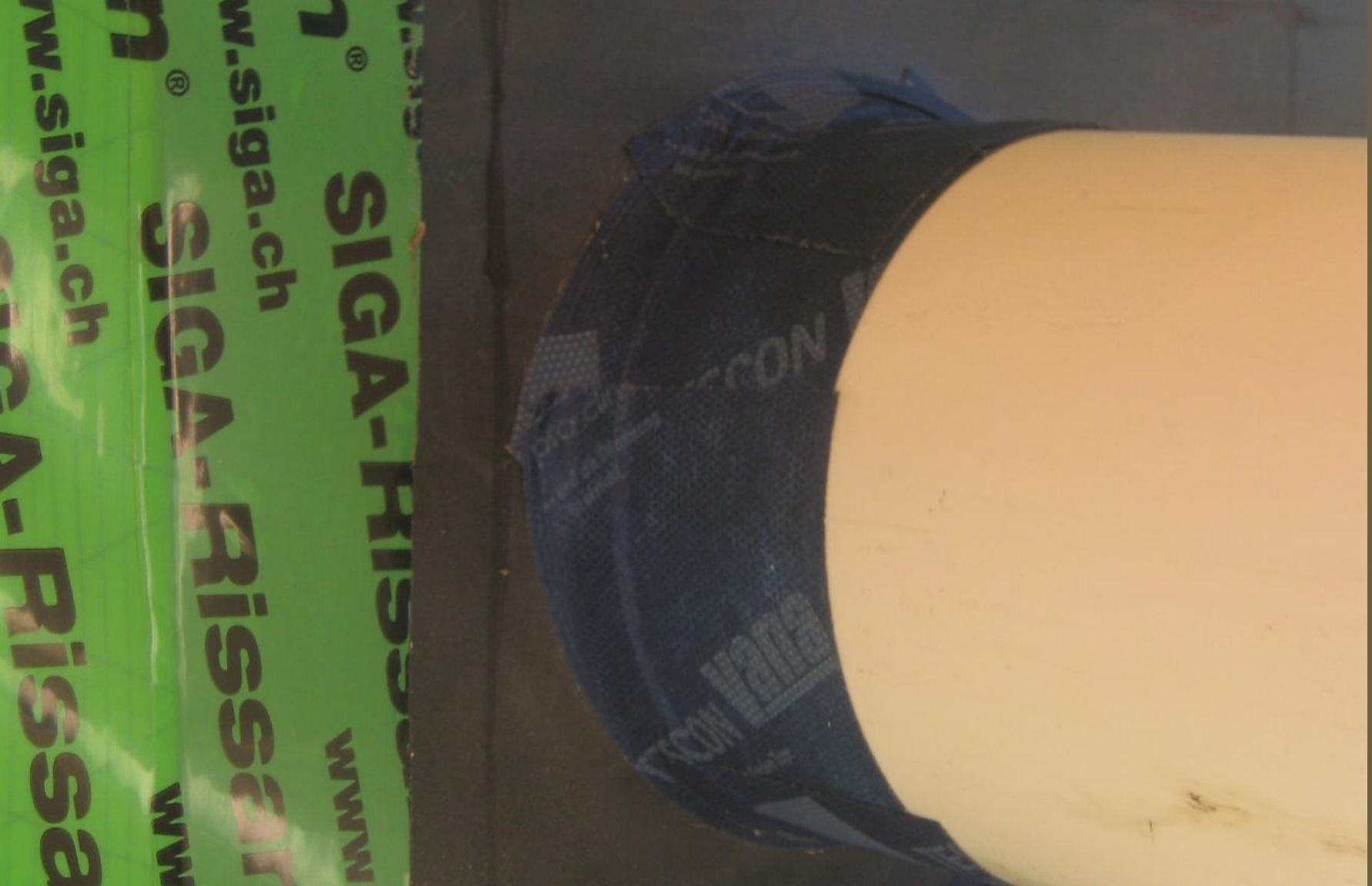
Gasket taping
