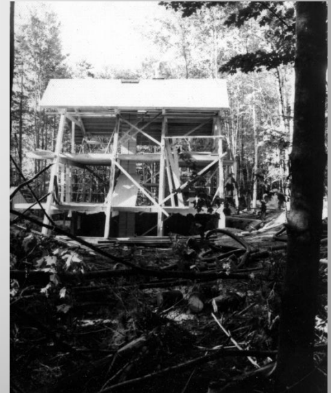
Green Lumber Framing
