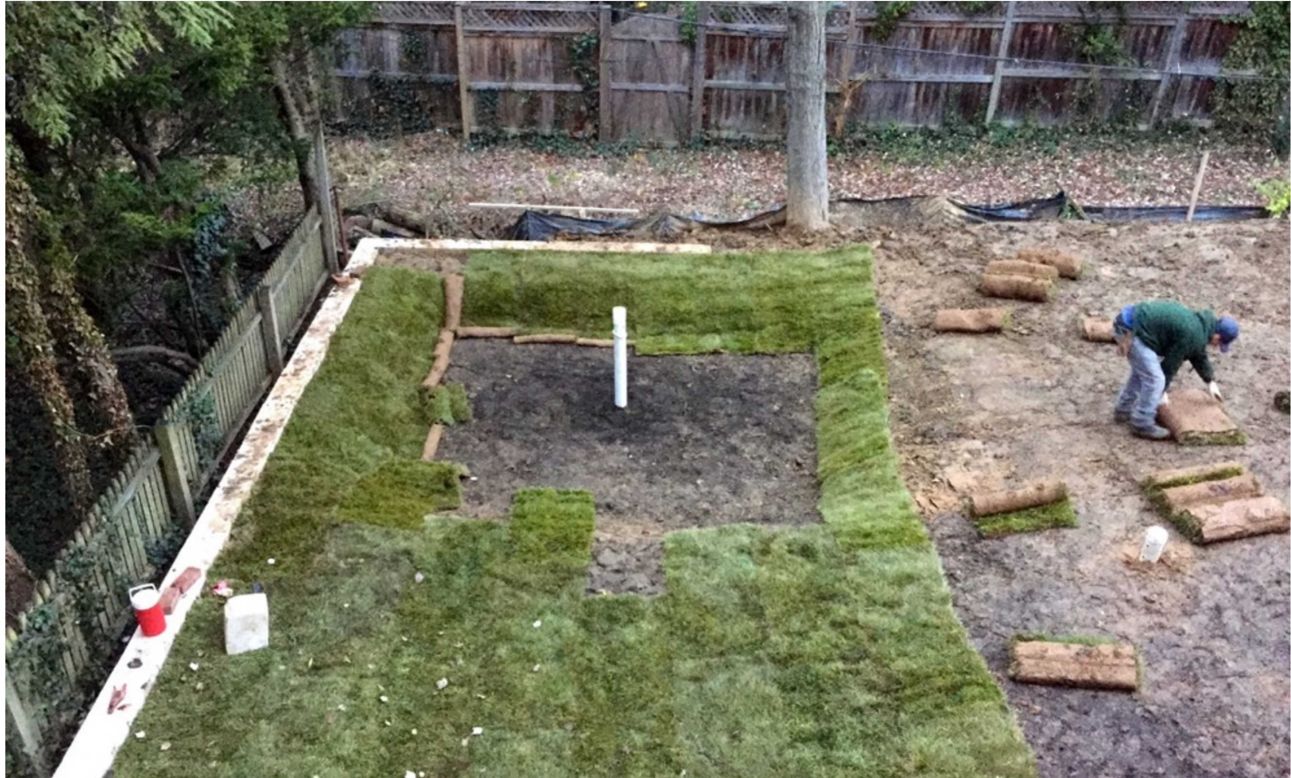
dry stacked AAC block retaining wall
