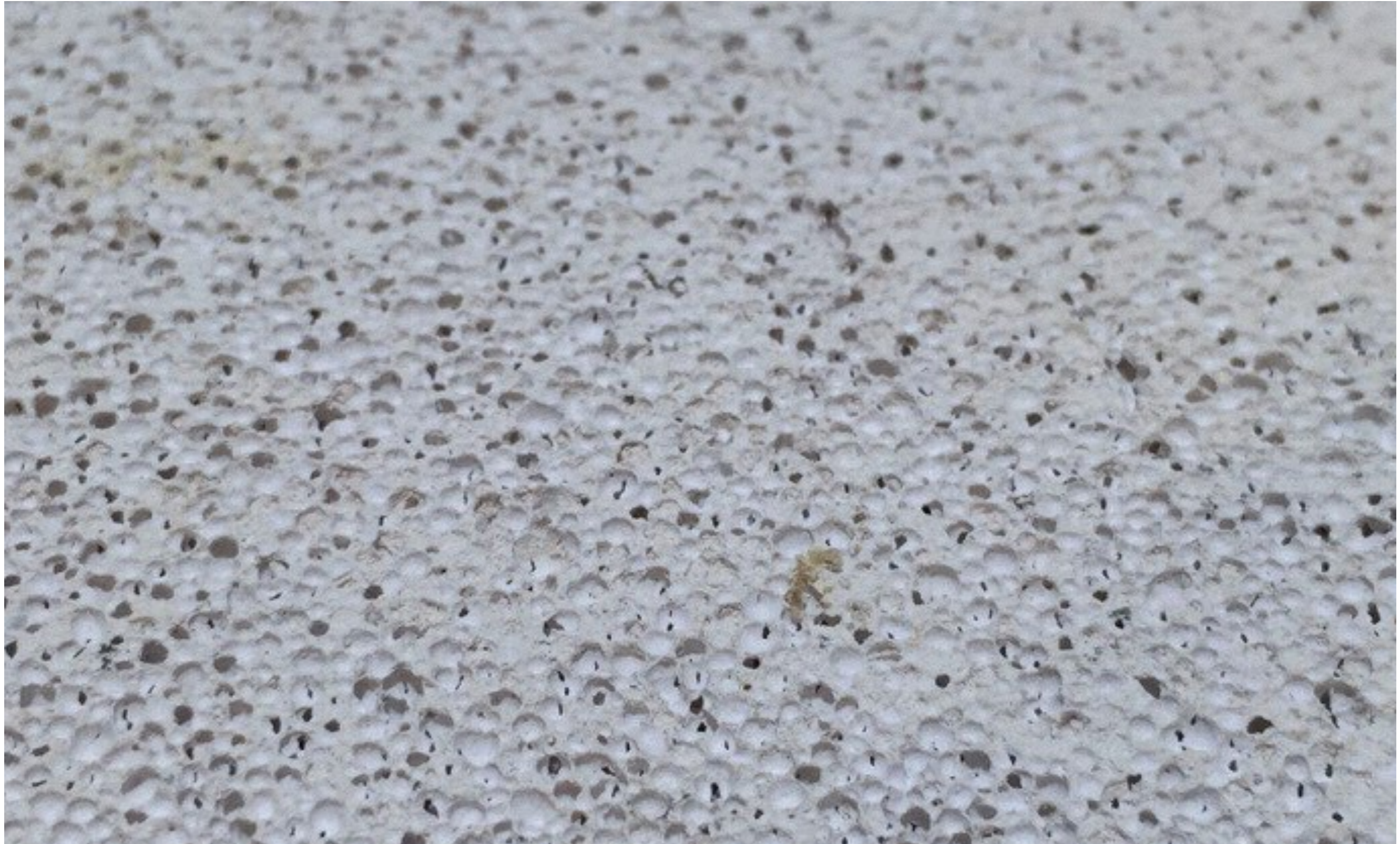
surface of autoclaved aerated concrete
