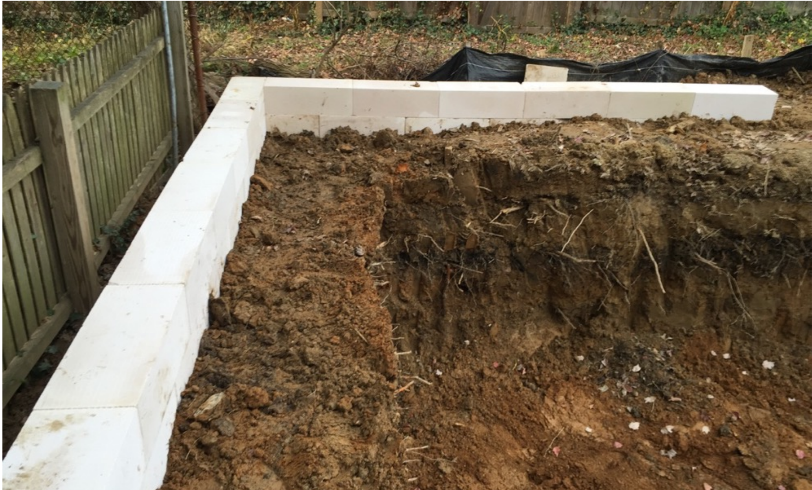
dry stacked AAC block retaining wall
