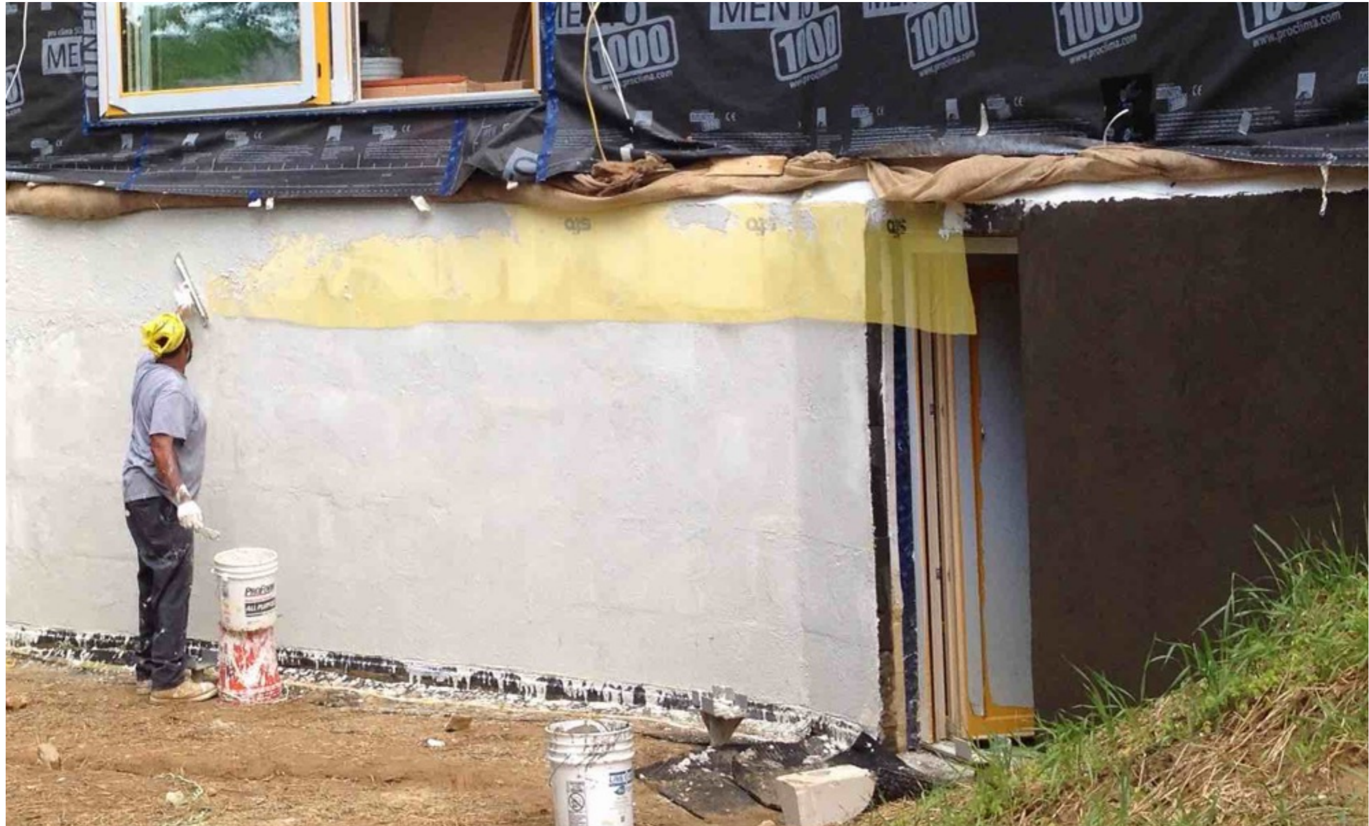
applying lime stucco
