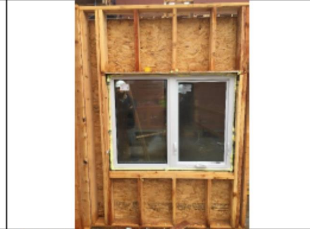
The installed window from inside.
