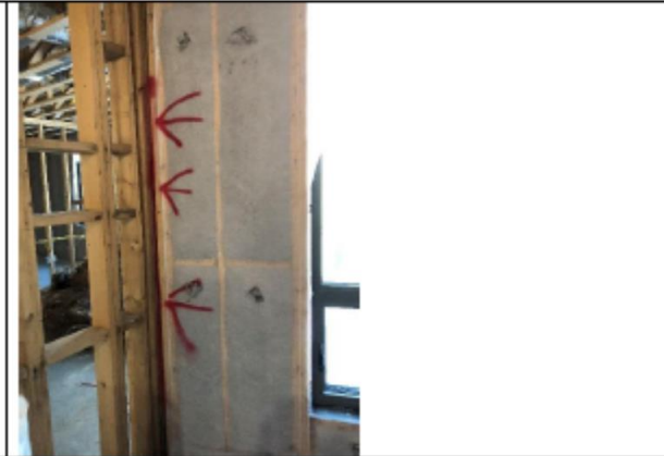
The installed window from outside. Locations where leaks were found are shown and described further below.
