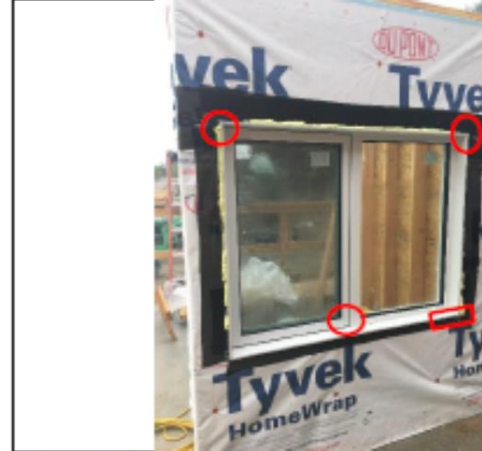
The installed window from outside. Locations where leaks were found are shown and described further below.
