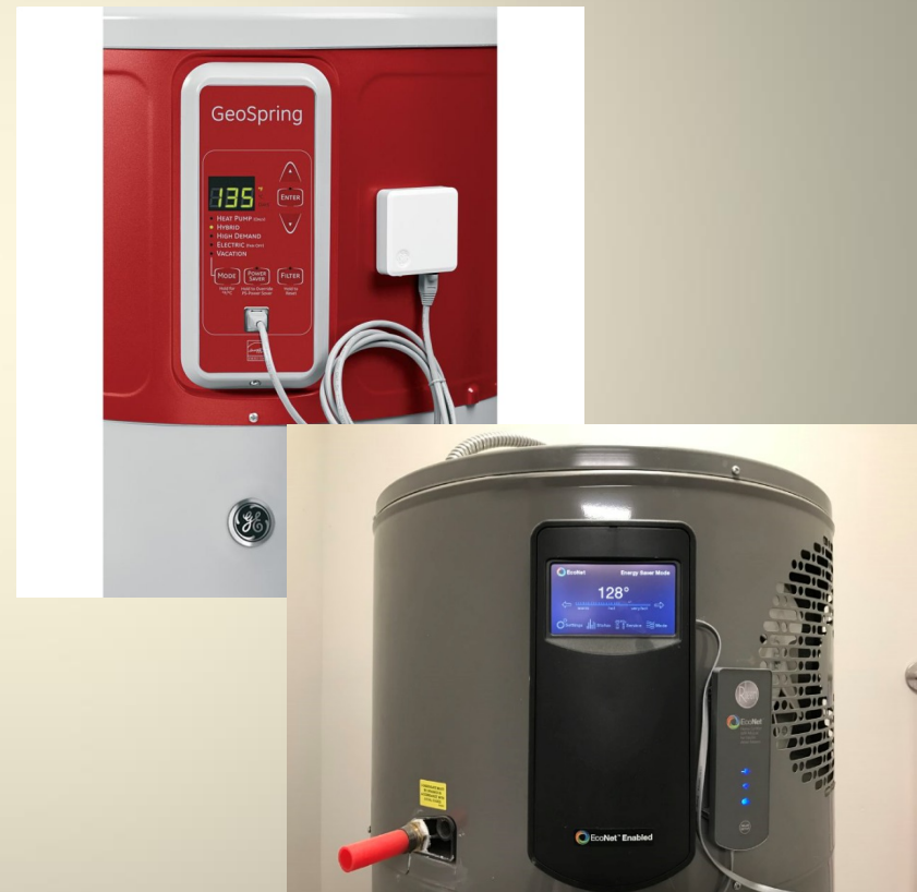
Heat Pump Hot Water (HPWH)
