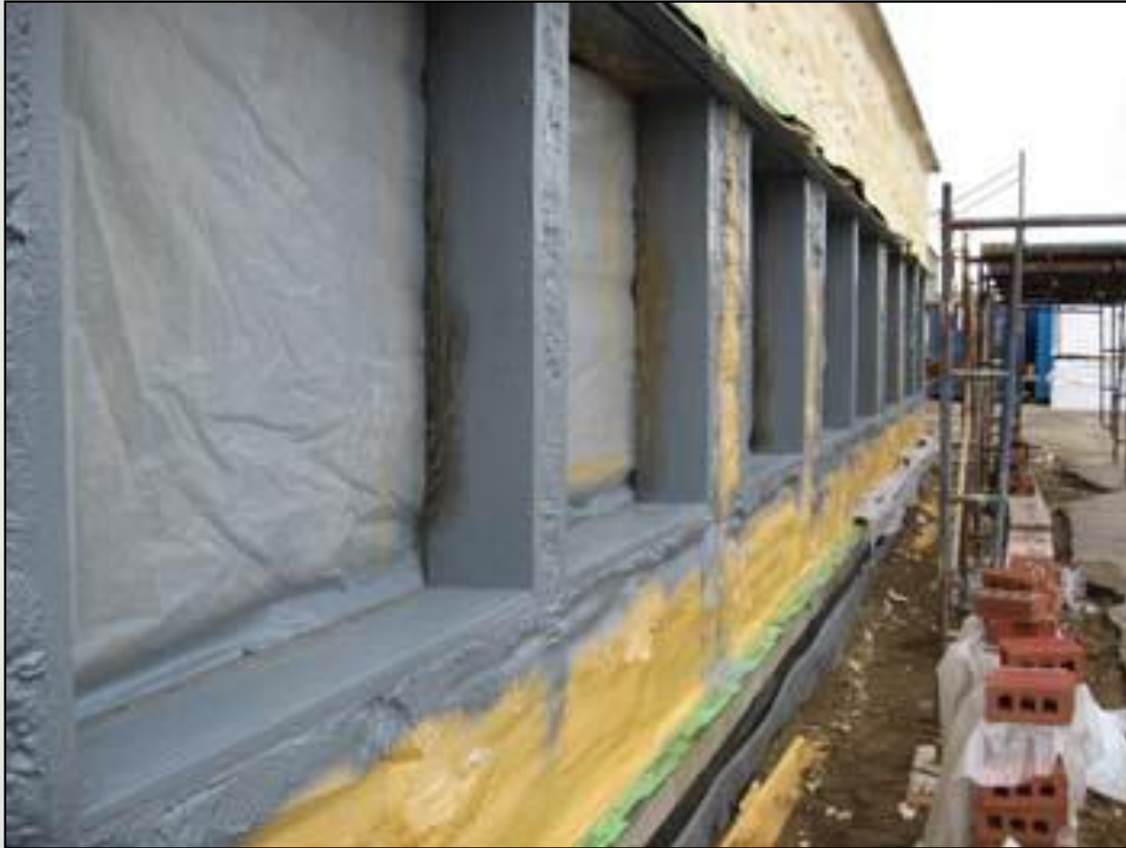
LAM application at multiple window openings
