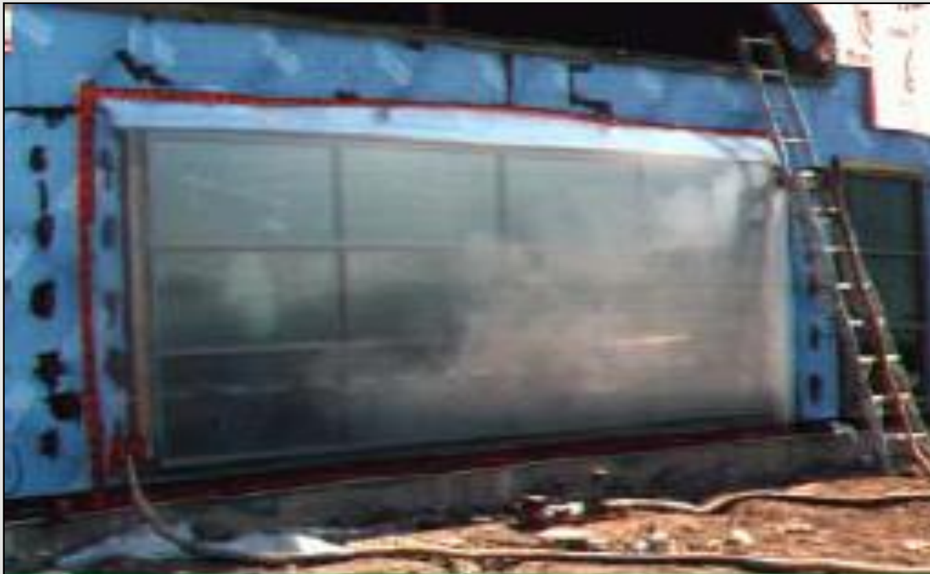
Figure 15: ASTM E 1186 4.2.6 smoke test being performed on a window.
