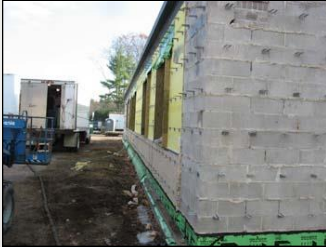
Masonry backup wall
