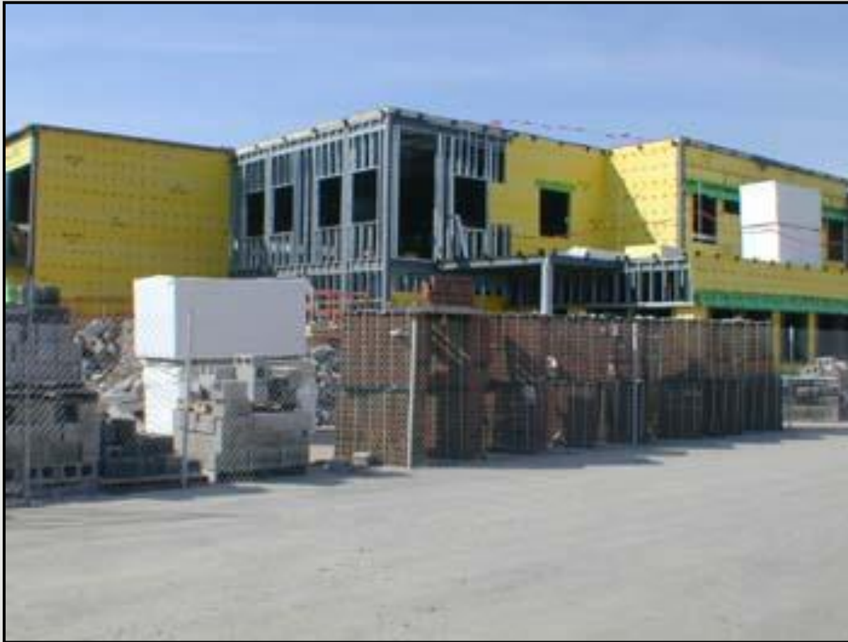
Metal stud and Densglas backup wall at new corner access addition
