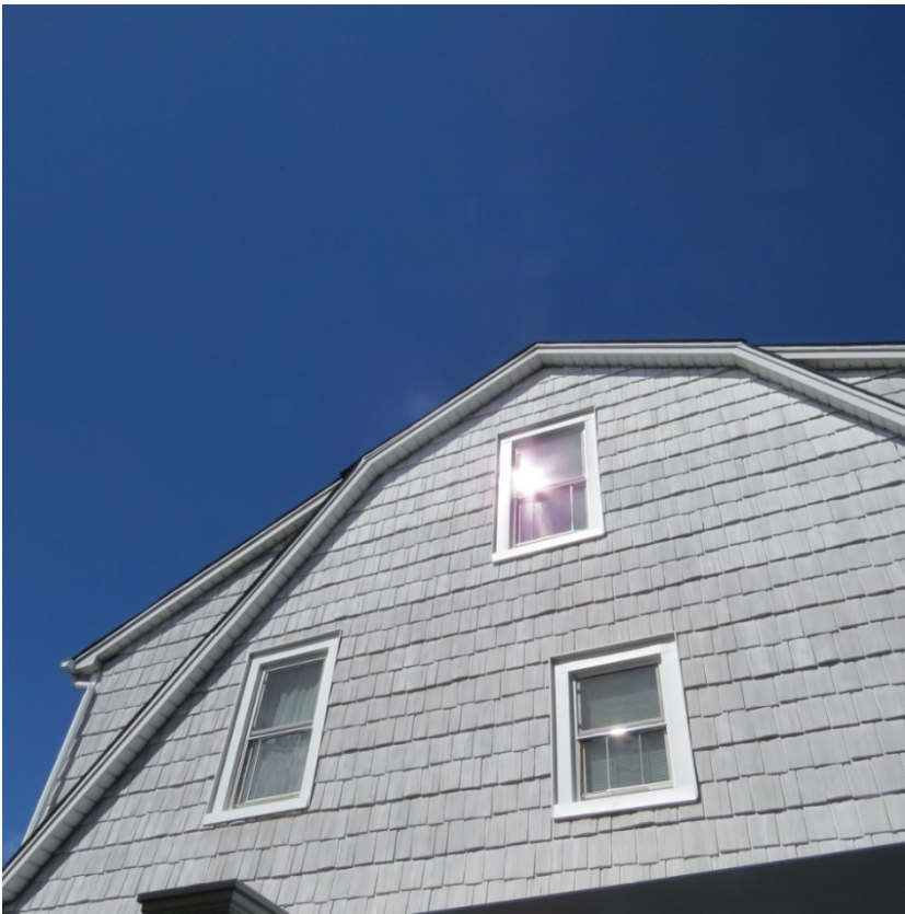
Solar Glare Reflection from Window
