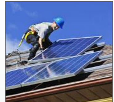
Conventional Rack-mounted Solar
