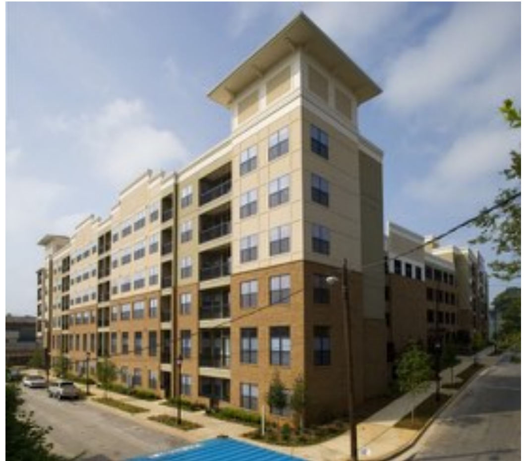
626 Dekalb Avenue, Atlanta, GA Matt Church - Davis Church Structural Engineers
